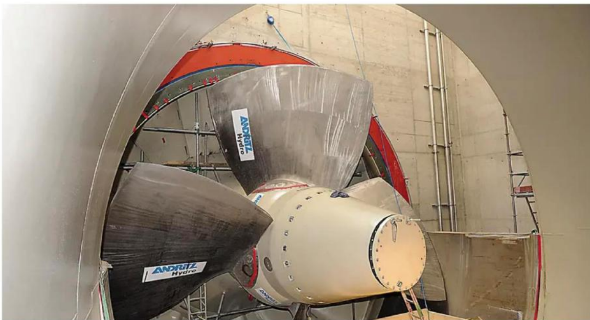
Bulb turbine runner during installation process at HPP Iffezheim, Germany
