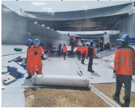
Figure 5. Lining Geomembran in Larona Hydropower
