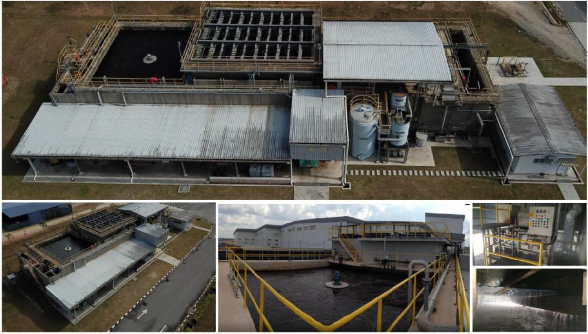
Figure 10. Waste water being treated and recycled in Waste Water Treatment Plant including washing sand filter, carbon filter, Beltpress machine, Static screen
