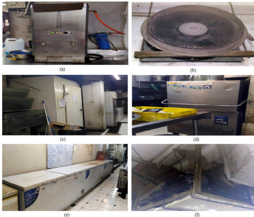
Figure. 1. Electrical Appliances at F&B Department: (a) Water heater, (b) Exhaust Fan, (c) Walk in chiller, (d) Dishwasher, (e) Under chiller, (f) Blower Wheel
