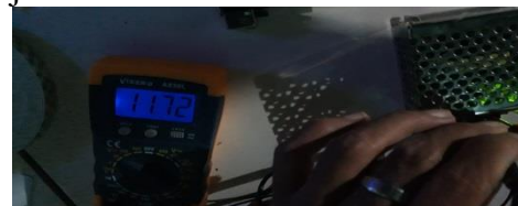
Gambar 4. 2 Power Supply 12VDC
