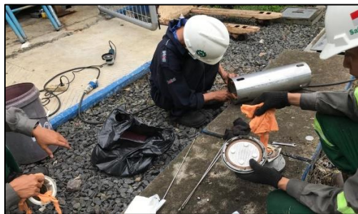
Gambar 6. Penggantian Filter Kompresor Kwangshin C-100
