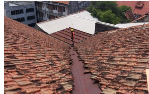
f. horizontal rainy gutter
