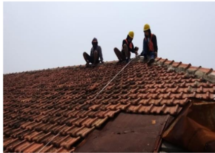
e. Roof and survey team
