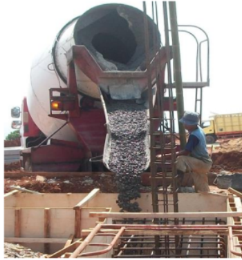
Foto 3: Gutter for casting concrete
