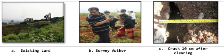
Figure 3 Survey of existing land and crack soil
