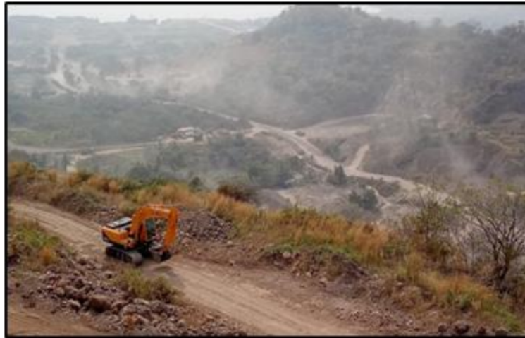
Fig 13. Excavator operational location
