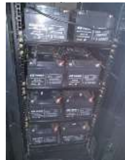
Gambar 6. Layout Battery UPS secara
