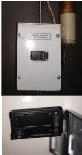
Gambar 4.3 Bagian Receiver Sensor Suhu
