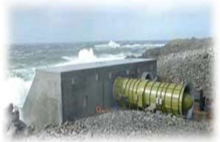
4. Bund Removed - Device Complete
