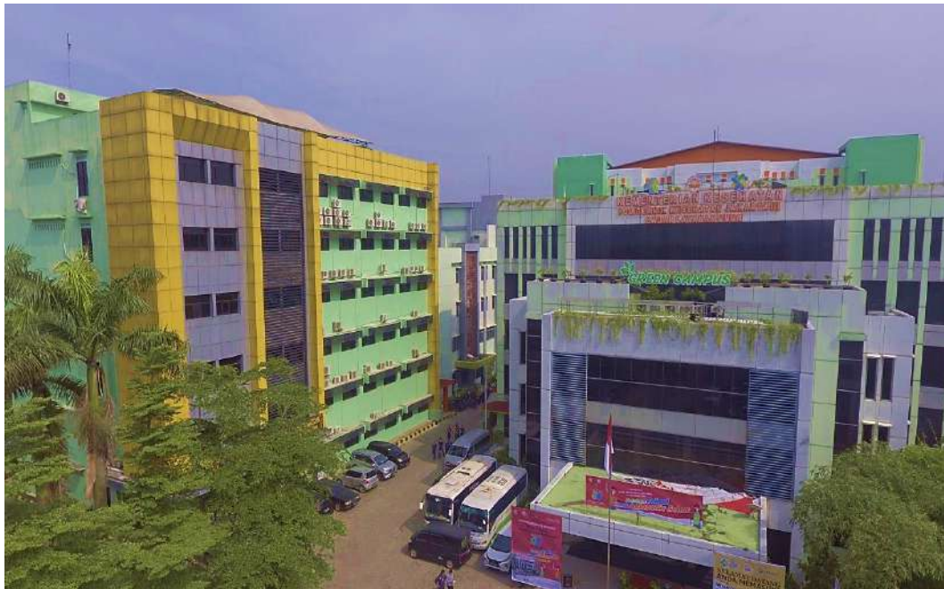
Gambar 1. Tampilan Gedung Poltekkes Kemenkes Jakarta III
