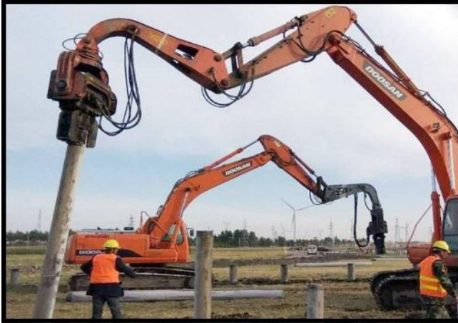
Gambar 3.4 Vibratory Pile Driver
