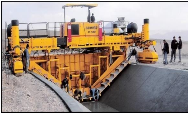
Gambar 1.22 Transverse Concrete Finisher
