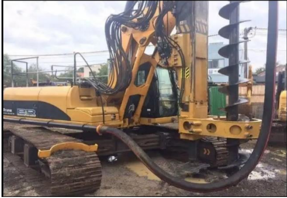
Gambar 3.8 Pile Boring Equipment
