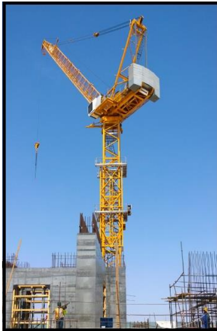
Gambar 2.12 Tied in crane
