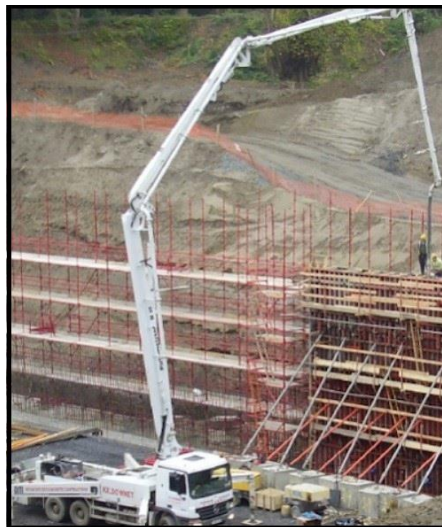
Gambar 5.5 Super Longboom Concrete Pump
