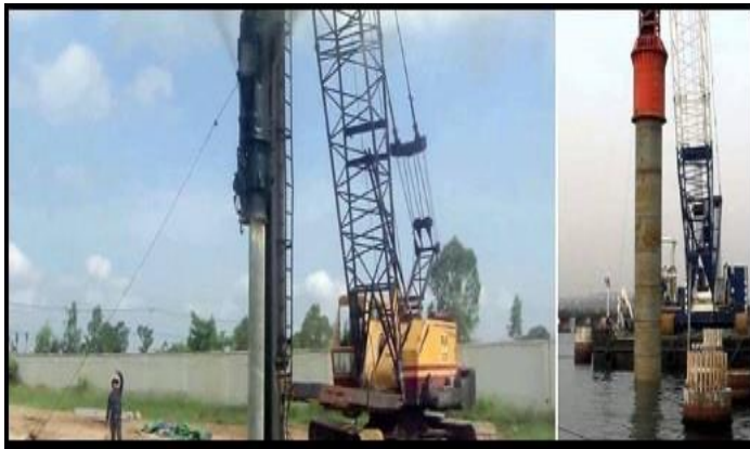
Gambar 3.2 Diesel Hammer
