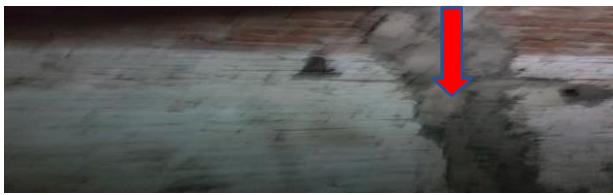
Figure 6. The wall of the 2 nd house cracked, covered with plaster(Source: Author document)
