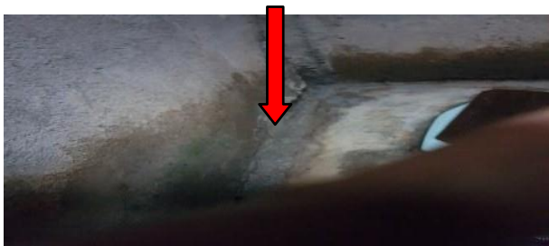
Figure 7. The wall of the 3 rd house cracked(Source: Author document)
